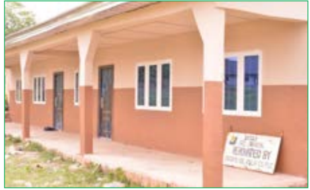
BLOCK OF THREE (3) CLASSROOM AT OKE COMMUNITY
